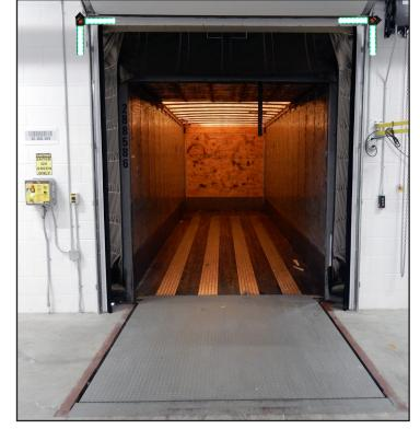
Mounted on the interior wall above the top two corners of the dock door, the lights extend out along the edges of the dock door opening to provide a visible indication when it's safe to enter the trailer.
