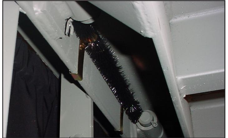
*When the brush is pressed into place it is supported by the metal clips. The brush expands sealing the void between the rear header and the hinge where air and rodents could enter.*
