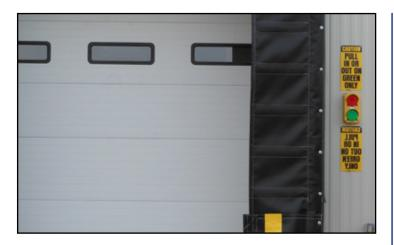
The outside lights can be paired with right reading and reverse reading signs to provide more communication with truck drivers.
